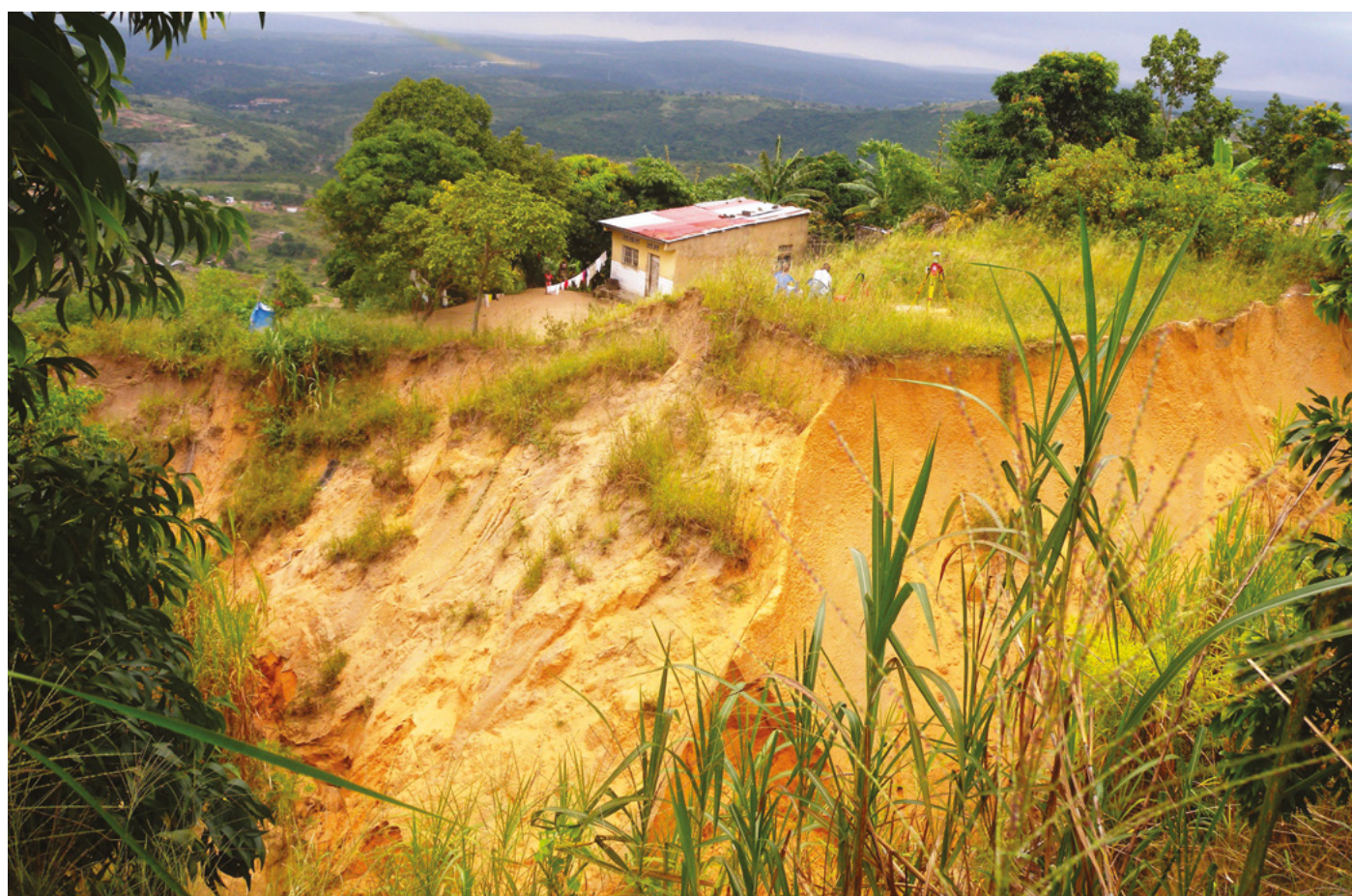
As gullies expand, they threaten people and community assets by destabilizing slopes and damaging buildings
