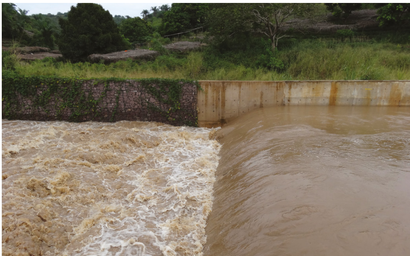
Intake point of the REGIDESO water treatment plant in Kimwenza. High level of sedimentation in the Lukaya River raises water production costs
