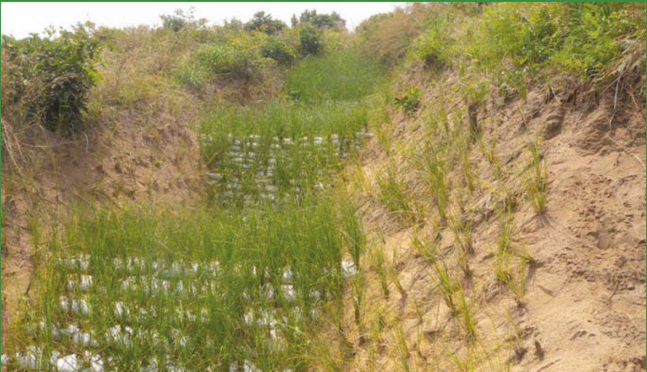
Gully stabilization in Mafumba using sandbags planted with vetiver grass: before (TOP) and after (BOTTOM) intervention.
