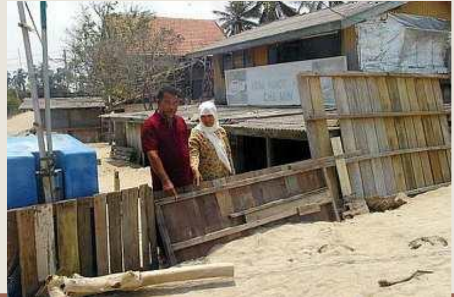
Makeshift Plank Wall Used as Wave Protection (March 2005)
