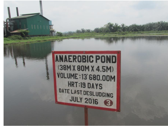
Primary Anaerobic Pond 3
