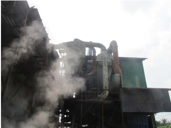
Shell & fibre used as boiler fuel
