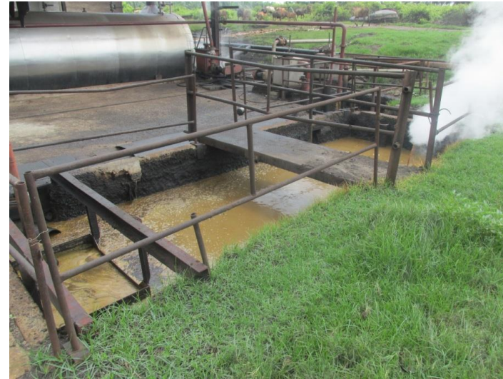
POME-Palm Oil Mill Effluent
