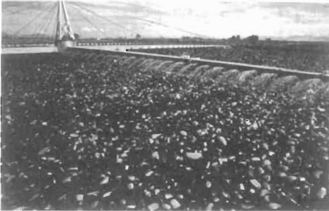
**Figure 9-11.** Trickling filter.
