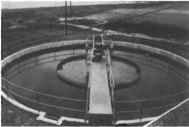
**Figure 9-7.** Circular settling tank.
