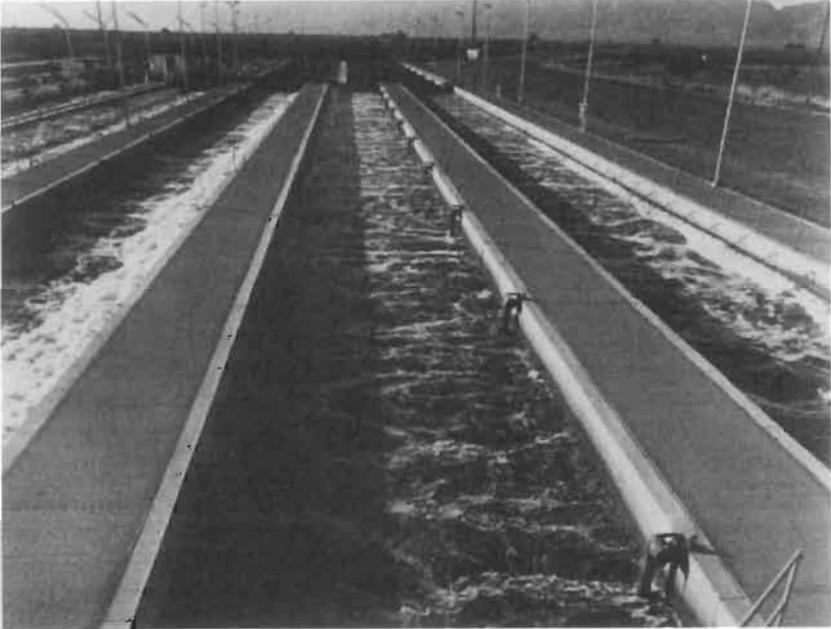
**Figure 9-15.** Activated systems with diffused aeration. (Photo courtesy of Envirex.)
