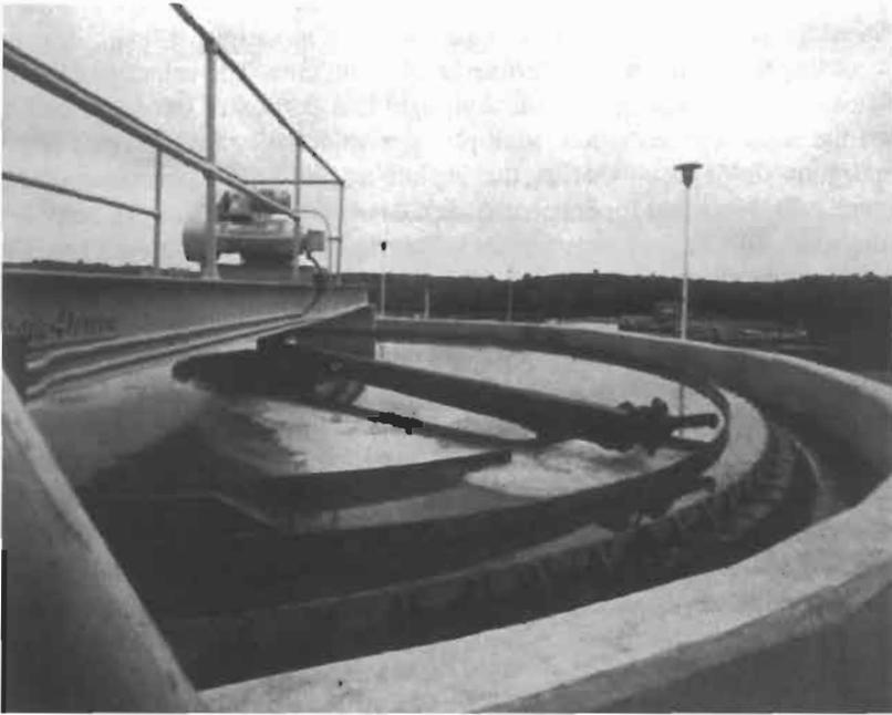
**Figure 10-6.** Gravity thickener. (Photo courtesy of Dorr Oliver Inc.)
