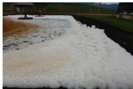
Plate ES-9 Foaming at aeration ponds in Pajam Landfill treatment process.
