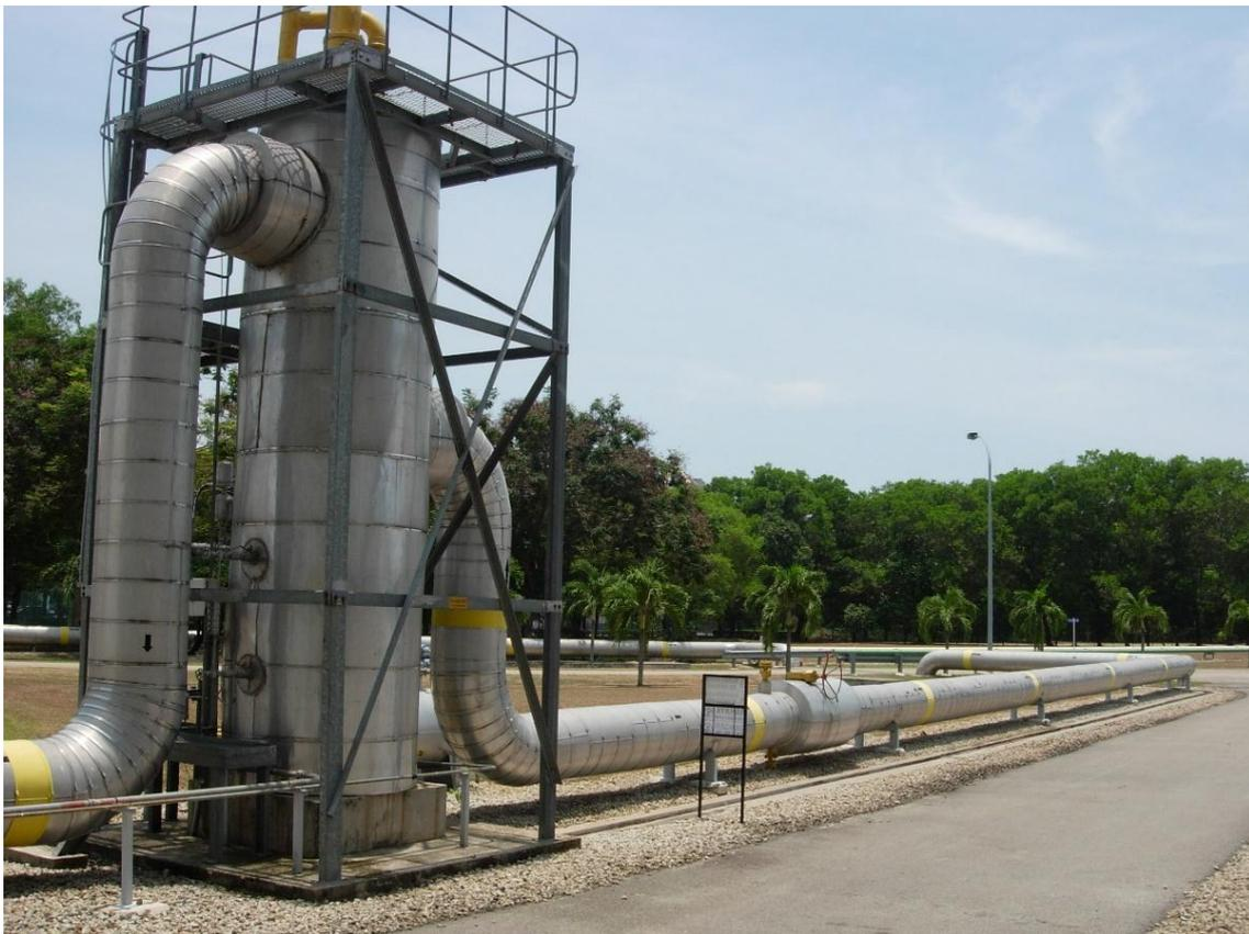
**Figure E-26: Example of gas pipes external lagging in industrial noise mitigation**
