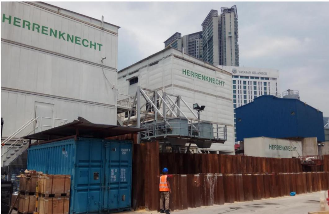
**Figure E-15: Full enclosure for slurry treatment plant in Klang Valley MRT construction work site adjacent sensitive receptors**
