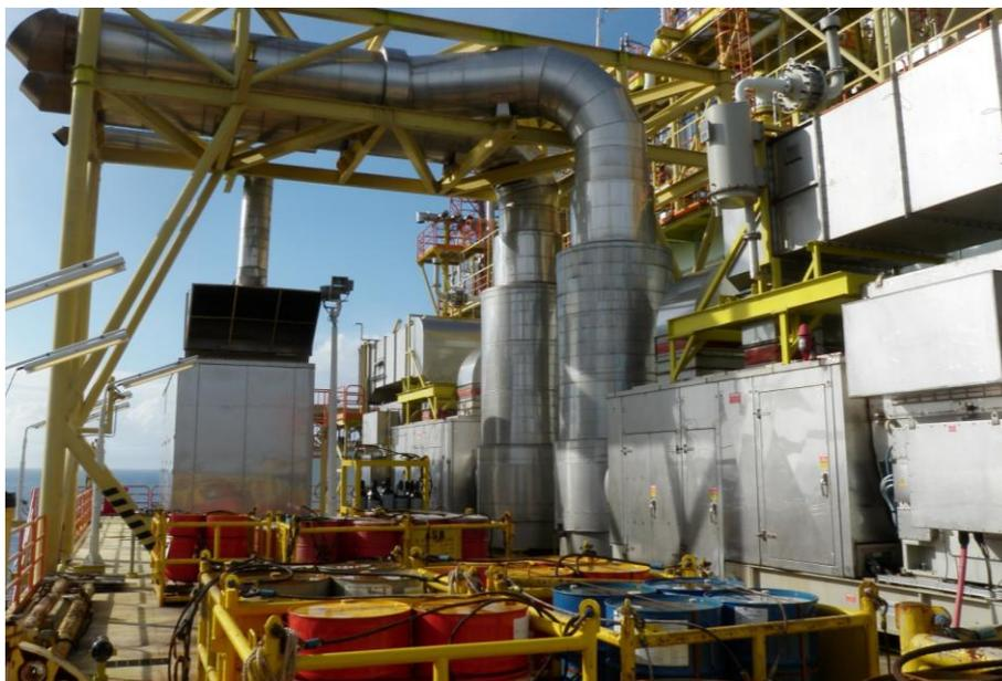
**Figure E-14: Full enclosure for power generating sets**
