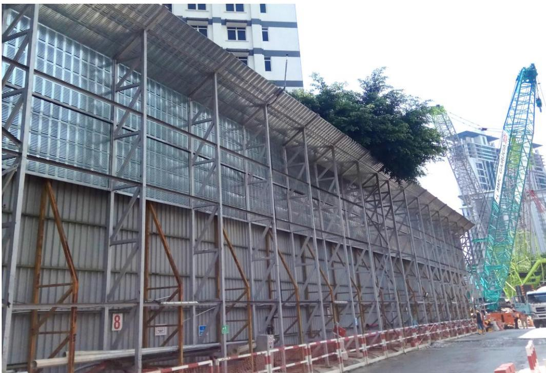
**Figure E-10: Temporary noise barriers used in MRT construction noise mitigation**
