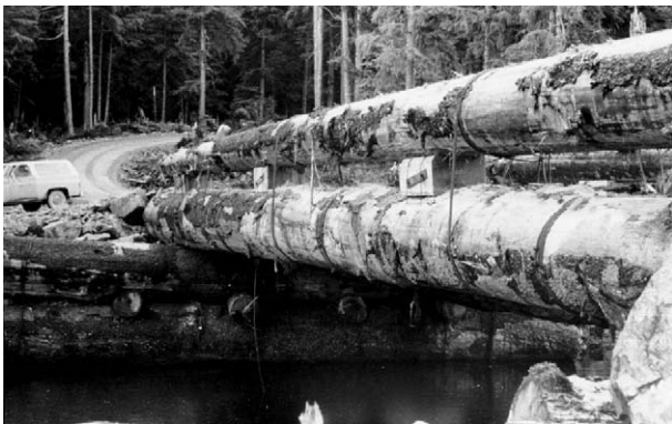
Figure 2 Logs are used to construct logging bridges in remote forest areas.
