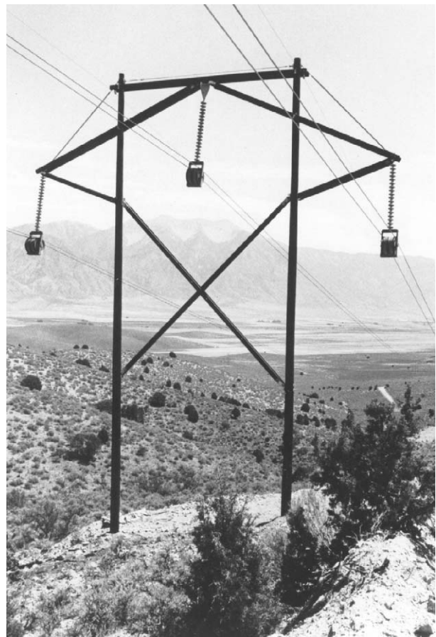
Figure 1 Round timber poles form the major structural element in these transmission structures. Courtesy of Koppers Co.
