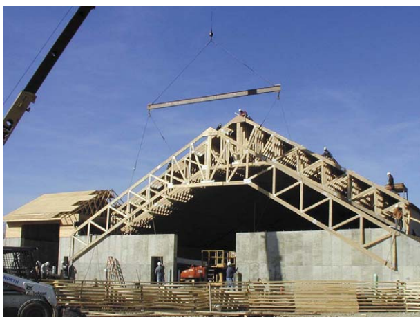
Figure 3 Roofs of virtually any shape can be framed with metal plate connected wood trusses fabricated from dimension lumber. Courtesy of the Wood Truss Council of America.
