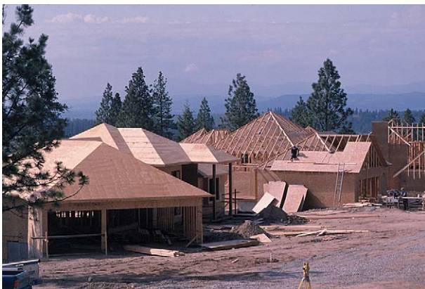
Figure 5 Light-frame buildings constructed from dimension lumber and plywood or oriented strand board sheathing such as these houses are the most common wood-frame structures. Courtesy of APA – The Engineered Wood Association.
