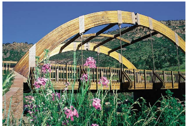
Figure 9 Hinged glue-laminated timbers support the deck of this graceful arch bridge. Courtesy of APA – The Engineered Wood Association.
