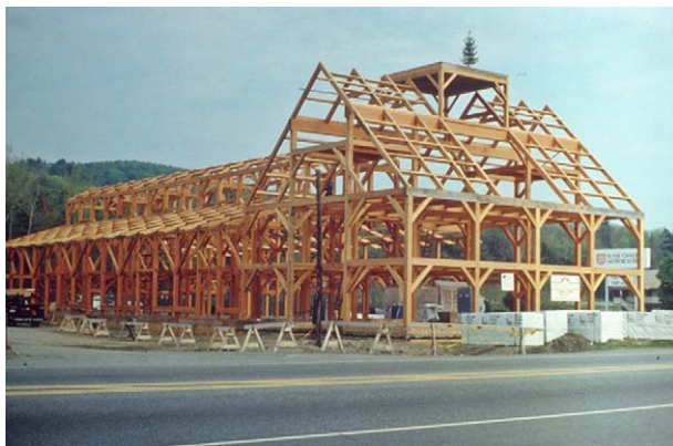
Figure 8 Diagonal braces lend rigidity to the timber frame of this future retail shop. Courtesy of Bensonwood Homes.
