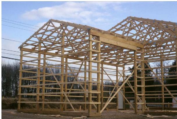
Figure 7 Diagonal bracing holds the dimension lumber walls and roof trusses of this post-frame building plumb and square before sheathing is applied. Courtesy of National Frame Builders Association.
