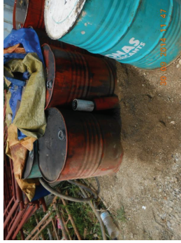
Plate 1b (Before): Contaminated sand is observed in the tray and no labelling (workers' camp).
