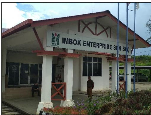
Plate 6.89: Imbok Estate site office
