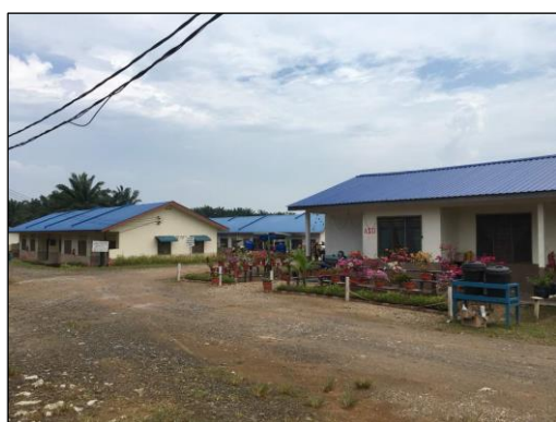
Plate 6.83: Samudera Estate workers' quarters
