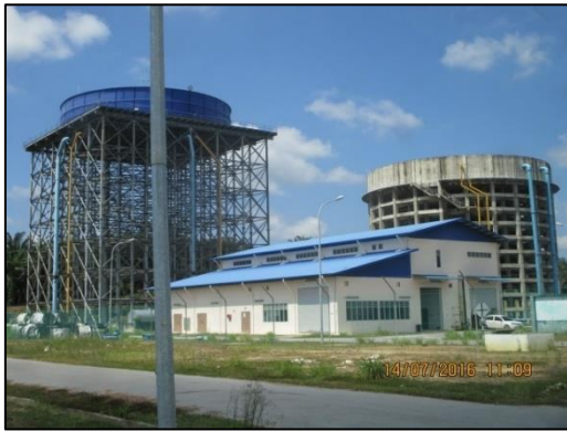
Plate 6.87: Samalaju water treatment plant
