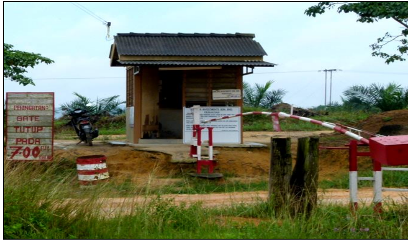
Figure 8-11: Example of Permanent Guard House
