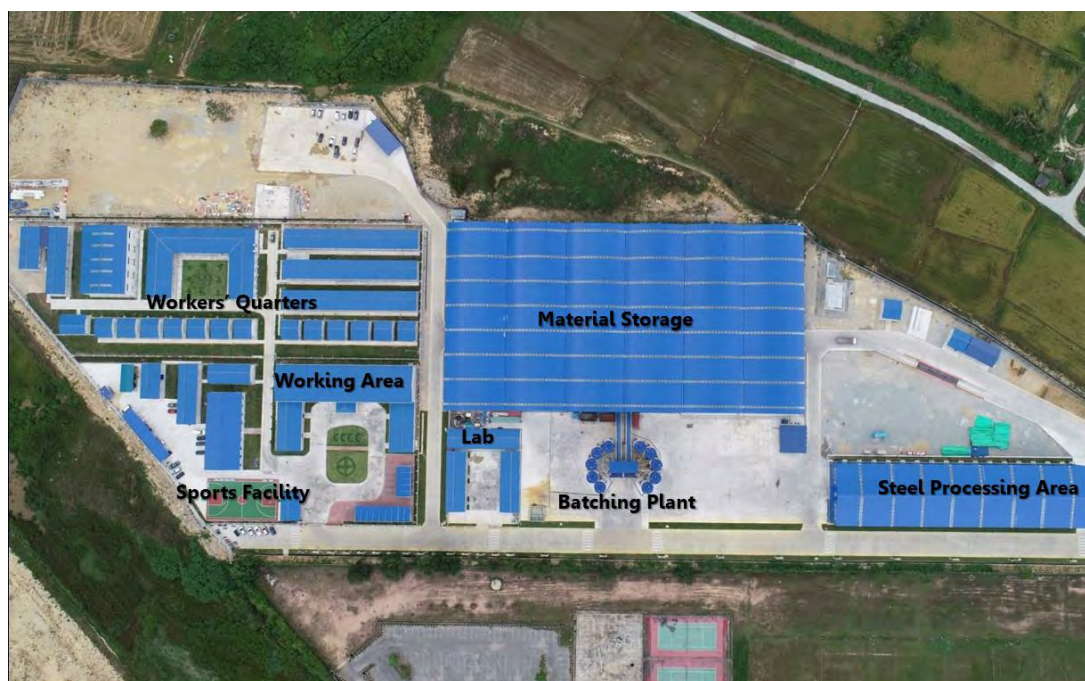
Plate ES-4 : Base Camp at Tunjong with Complete Facilities including Workers Quarters
