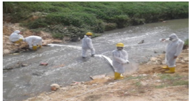
Kerja-Kerja Pemasangan Boom di Sungai Kim-Kim Boom Installation at Kim-Kim River
