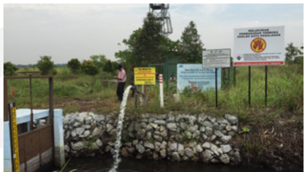
Kombinasi Menara Tinjau, Telaga Air Tanah, Sekatan Saliran dan Papan Tanda Larangan Pembakaran Terbuka di Kuala Langat, Selangor Combination of Tube Well, Check Dam, Watch Tower and Open Burning Prohibited Sign at Kuala Langat, Selangor
