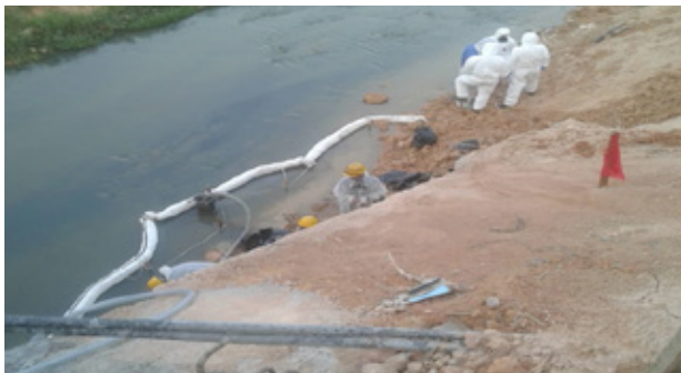
Kerja-Kerja Pemasangan Boom di Sungai Kim-Kim Boom Installation at Kim-Kim River
