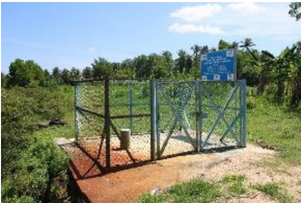
Paip Saluran Air di Hutan Simpan Raja Musa, Kuala Selangor, Selangor bagi Meningkatkan Paras Air Tanah Gambut Water Pipeline in Raja Musa Forest Reserve, Bestari Jaya, Selangor to Raise Peat Land Water Level
