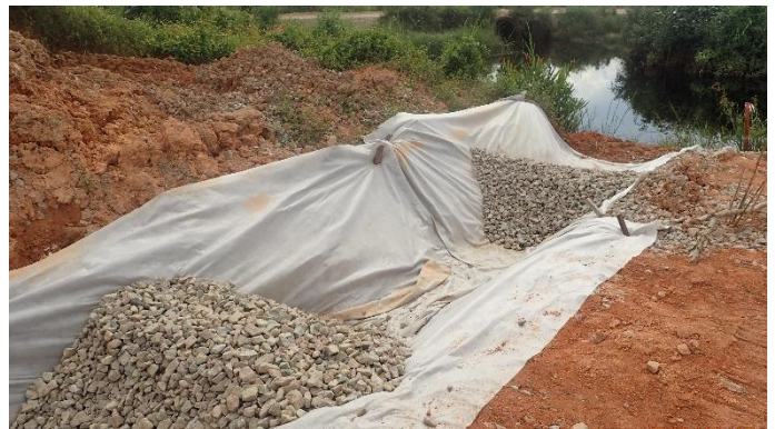
Temporary silt trap
