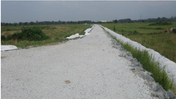
Access road covered with crusher run
