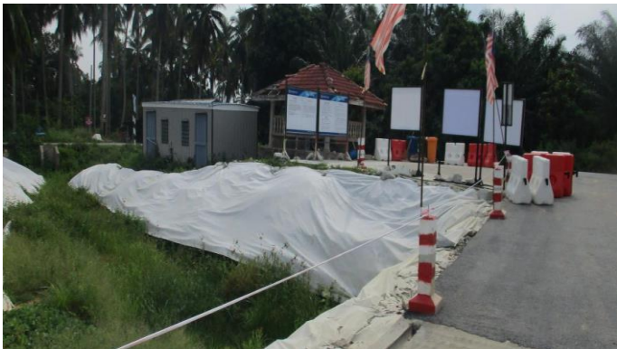
Slope covered with geotextile fabric (ii)
