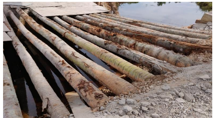
Biomass reused as temporary bridge
