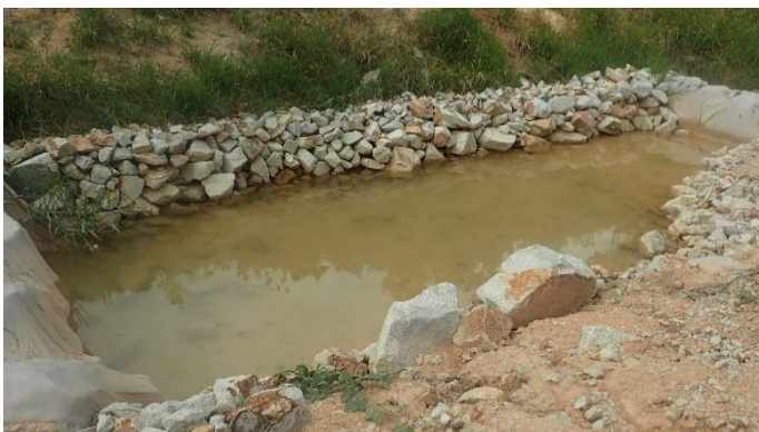
Silt trap with riprap protection
