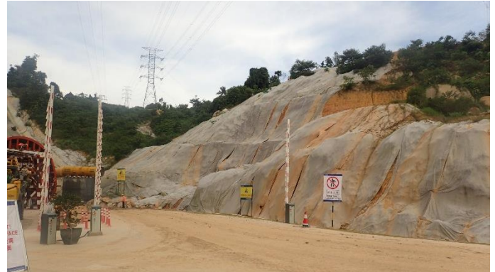
Slope covered with geotextile fabric (i)
