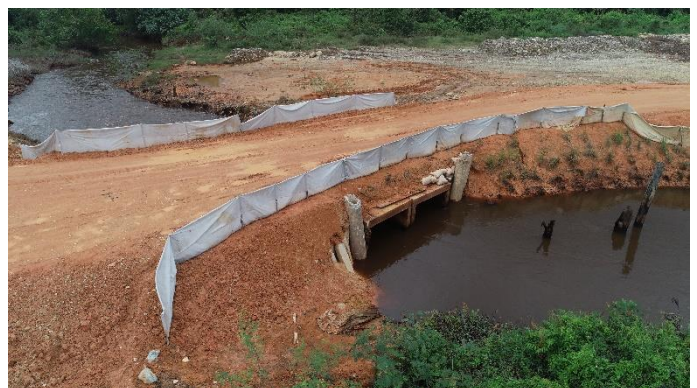
Silt fence at road crossing
